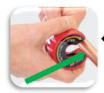
Mark where you want to cut on tube and insert the cutter.
